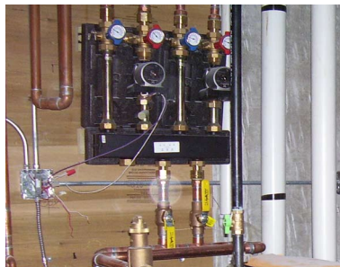
Concrete Home Naperville Illinois
